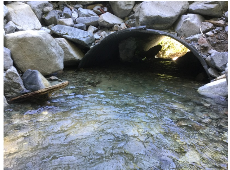
Looking through culvert from inlet
