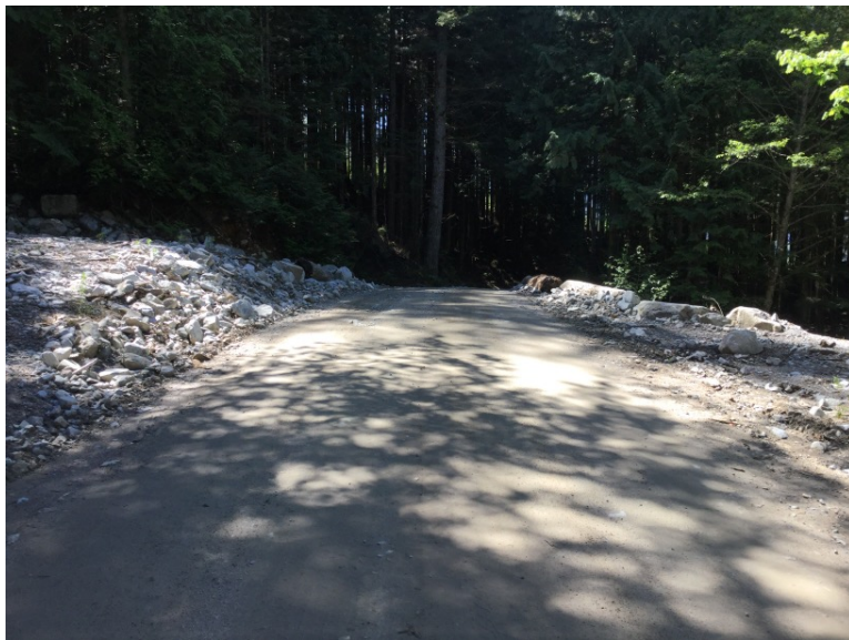
Approach from Right Bank when facing downstream
