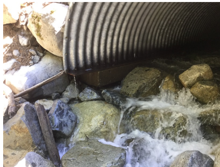
Footings exposed at outlet - right bank shown
