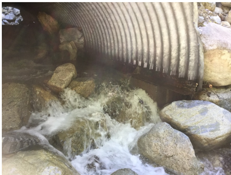
Footings exposed at outlet - left bank shown
