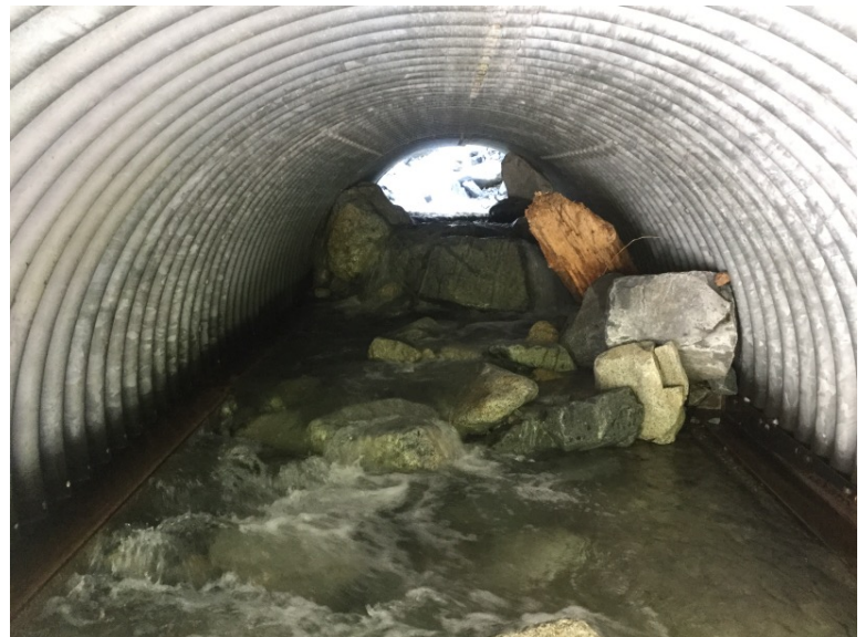
Looking through culvert from outlet
